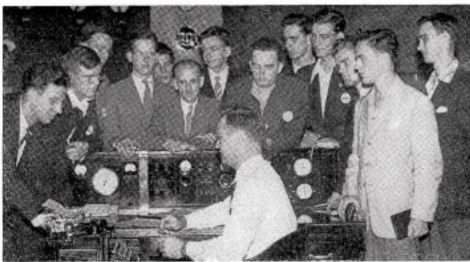
INSPECTING the control panel of the WJZ transmitter at Bound Brook, N. J., are the 11 finalists competing in RCA's nationwide contest for a $4,000 scholarship to the boy best equipped for a scientific career in wireless engineering [winner, fourth from right]. Seated at the desk is D. M. Stair, control engineer, while Engineers John Gullans (at extreme left), and Henry Steger (standing opposite Stair), explain the details.
